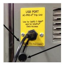
The breaker trip unit is connected to a receptacle on the breaker cubicle door.
